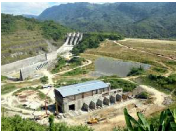
Bird's eye view of Power House, Spillway & Dam
