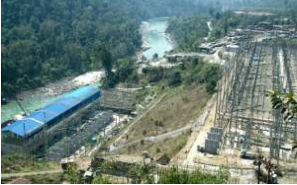
Bird's eye view of Power House
