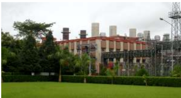
Assam Gas Based Combined Cycle Power Plant, Assam
