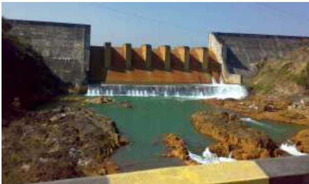
Kopili Hydro Electric Plant, Assam
