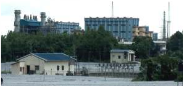
Solar PV Power Plant at TGBP Site, Tripura
