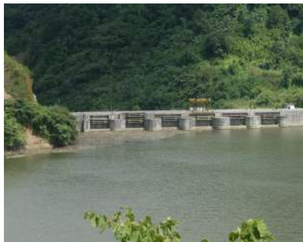
Ranganadi Hydro Electric Plant, Arunachal Pradesh
