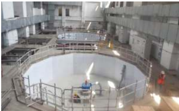
Power House inside view
