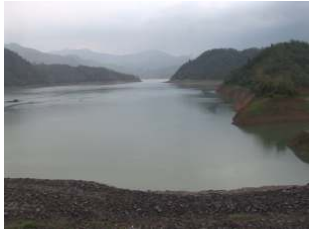
Doyang Hydro Electric Plant, Nagaland
