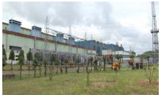
Agartala Gas Based Combined Cycle Power Plant, Tripura
