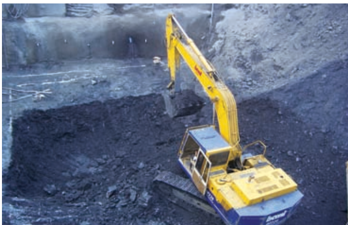
Work in progress at Kameng HE project
