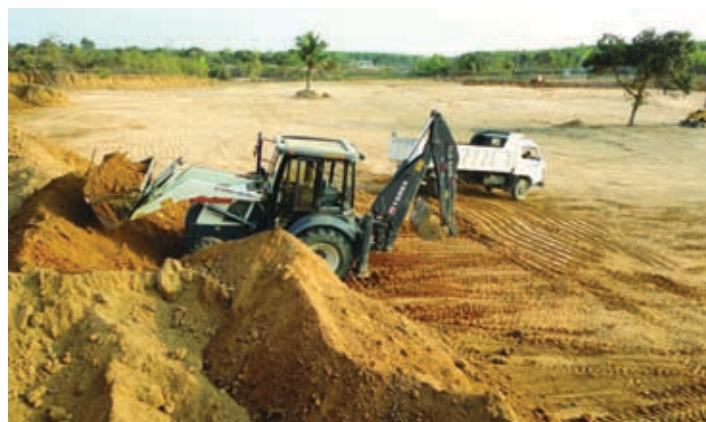
Site levelling works in progress at TGBPP
