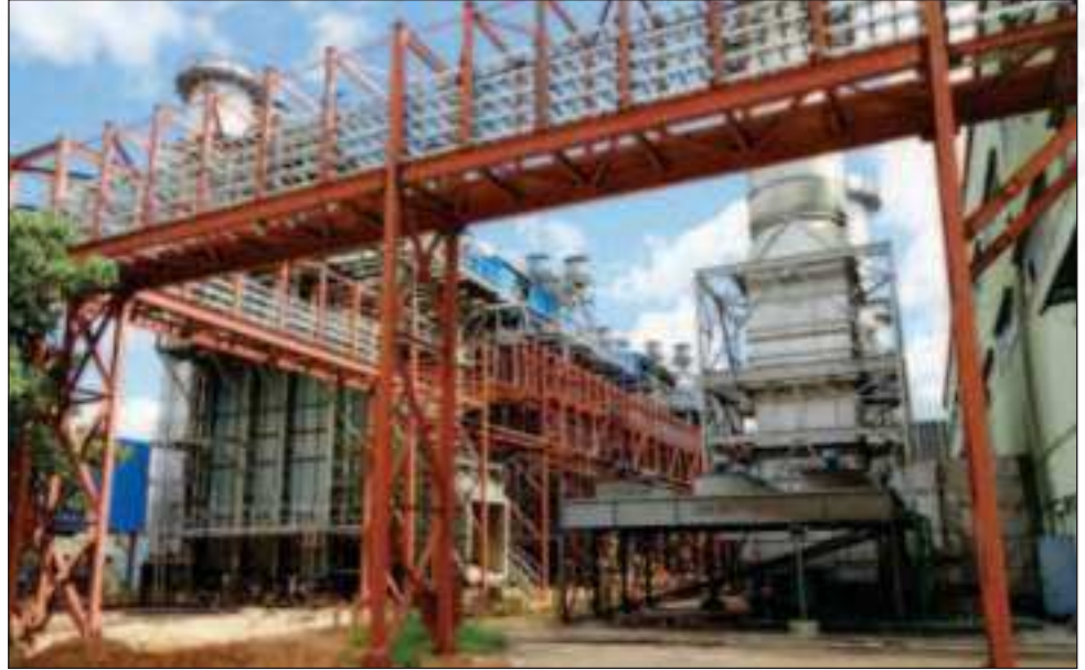
Agartala Gas Turbine Plant- Combined Cycle Extension Project
