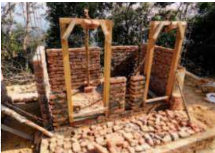
School toilets in progress at wokha Nagaland
