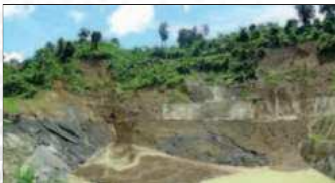
Power House site, Tuirial Hydro Electric Project
