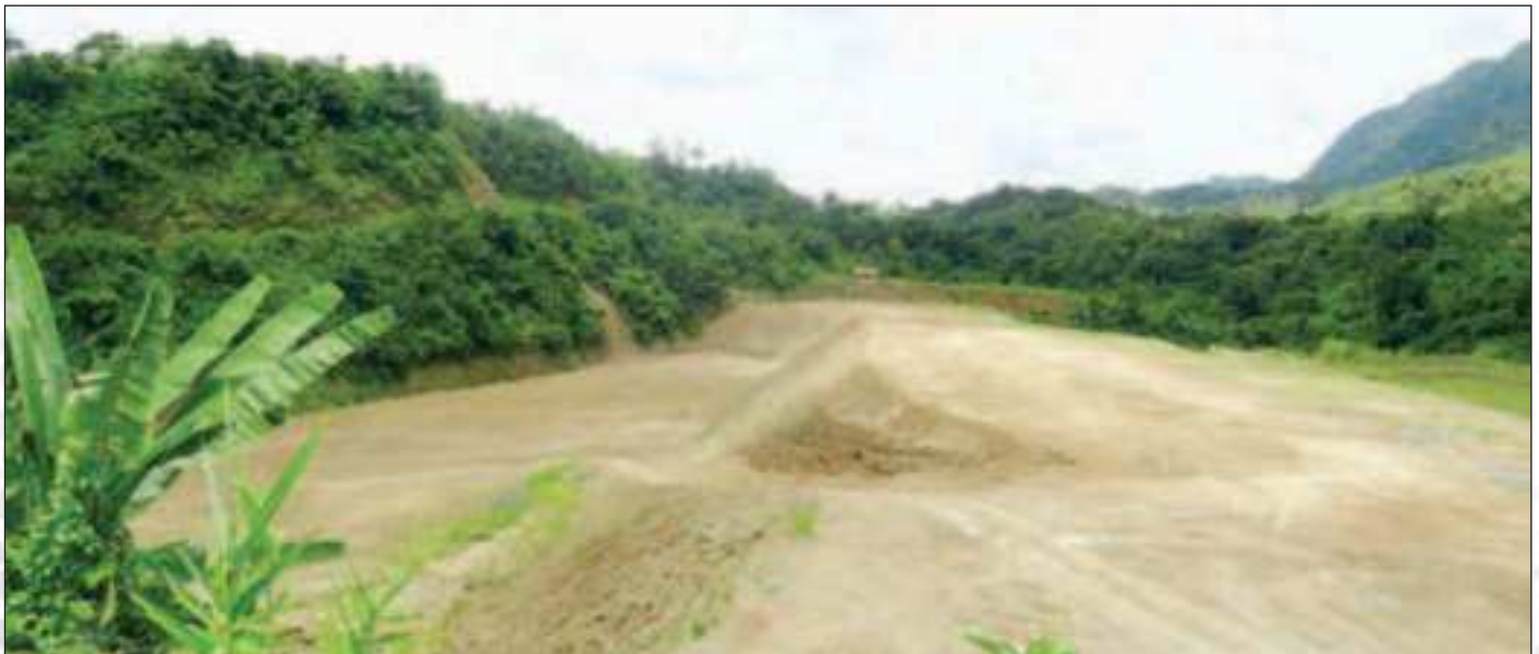
Upper Coffer Dam, Tuirial Hydro Electric Project
