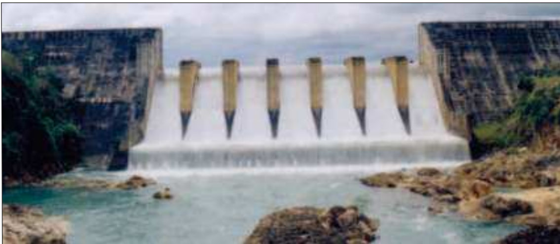
Kopili Hydro Electric Plant
