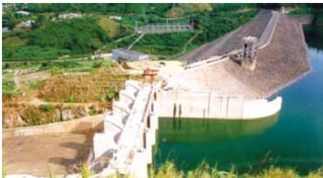
A view of dam and spillway, Doyang Hydro Electric Plant
