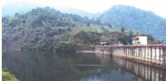
Ranganadi Hydro Electric Plant
