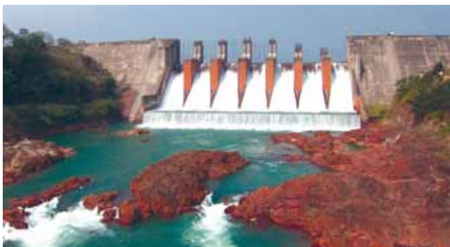
Kopili Hydro Electric Plant
