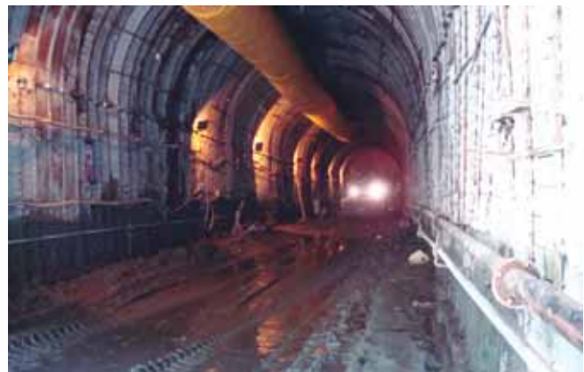
Completion of Afrit - I (Pare HEP)
