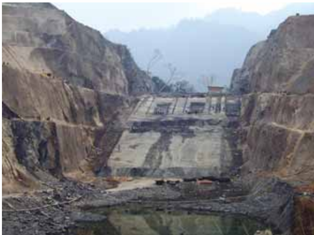
Work in progress at TrHEP
