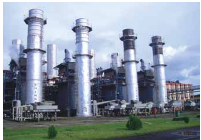
Chimney at AGBP
