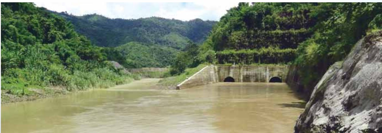
Downstream Cofferdam, Tuirial Hydro Electric Project
