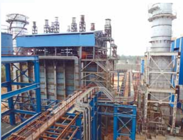
Tripura Gas Based Project Power House under construction
