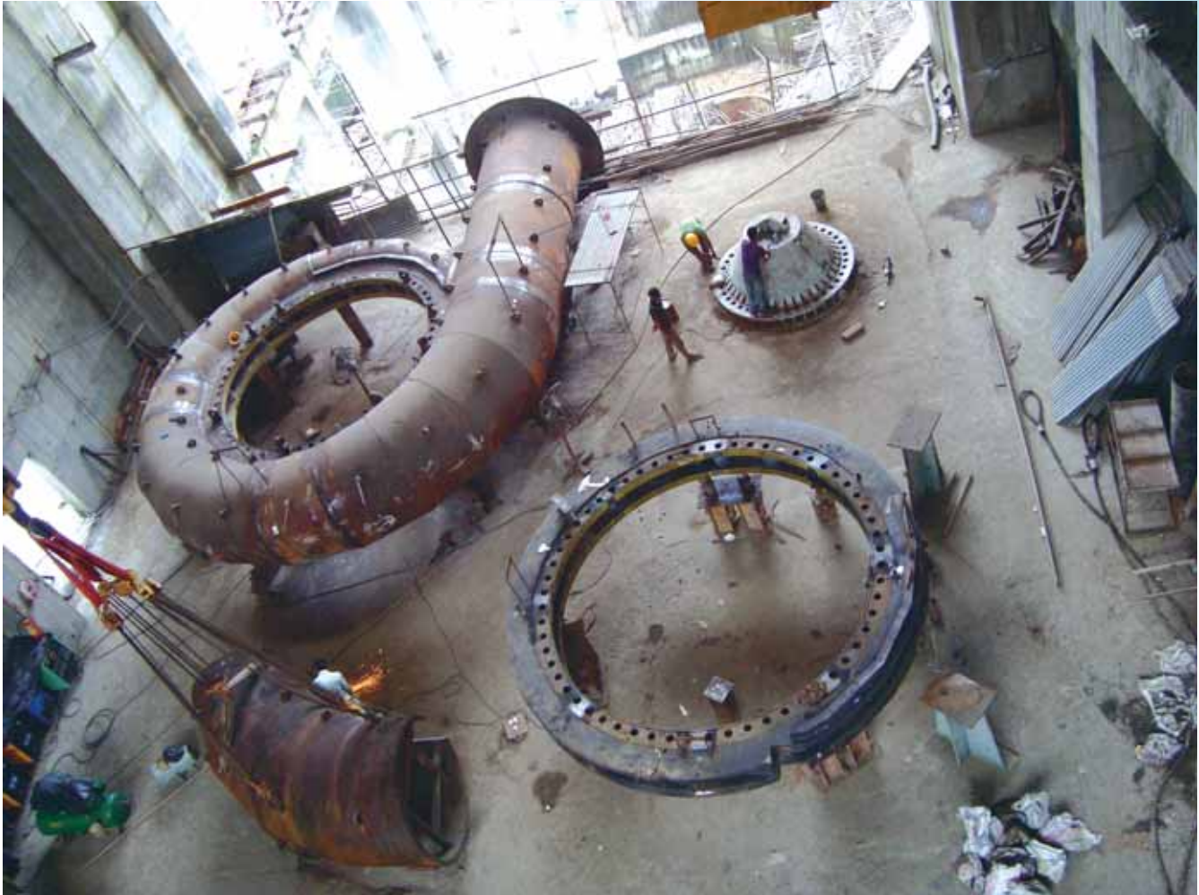
Work in progress at Kameng Hydro Electric Project
