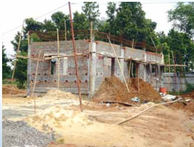
Inverter Room No. 1 under construction at the Solar Power Project, Monarchak
