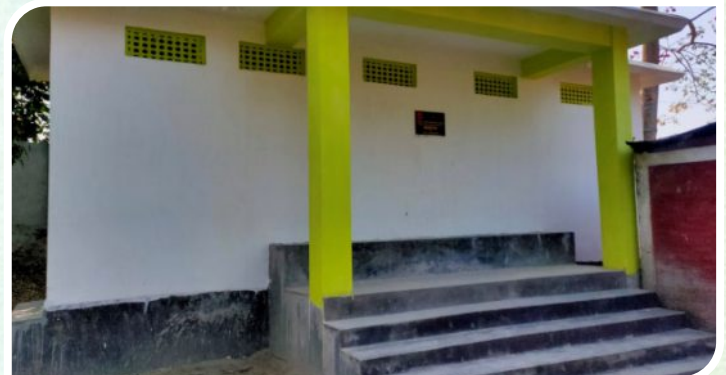
Construction of Toilet and attached waiting shed in the premises of No.-1 Kamalabari L.P. School, Majuli District, Assam.
