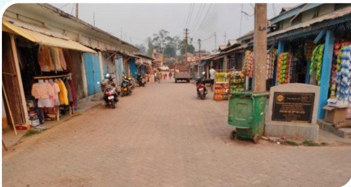
Construction of Road concrete block at Umrongso Market, District - Dima Hasao, Assam
