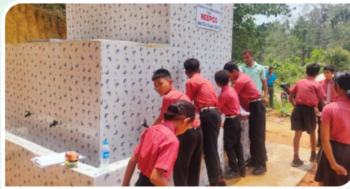
Construction of Drinking Water filter Tank for Gaya Charan Memorial International School, Gachia Para, Tripura (W)
