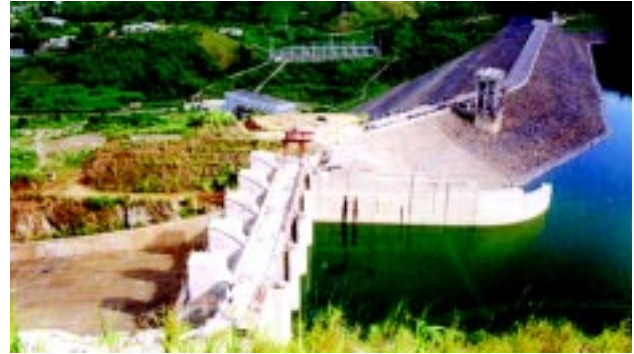
A view of the dam and spillway, DHEP, Nagaland
