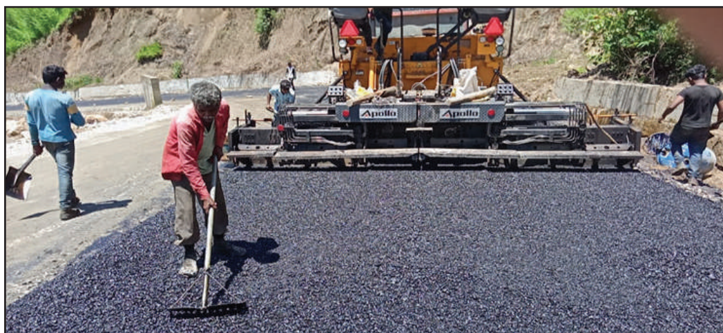
Ongoing Project Joram-Koloriang Pkg-3, Arunachal Pradesh
