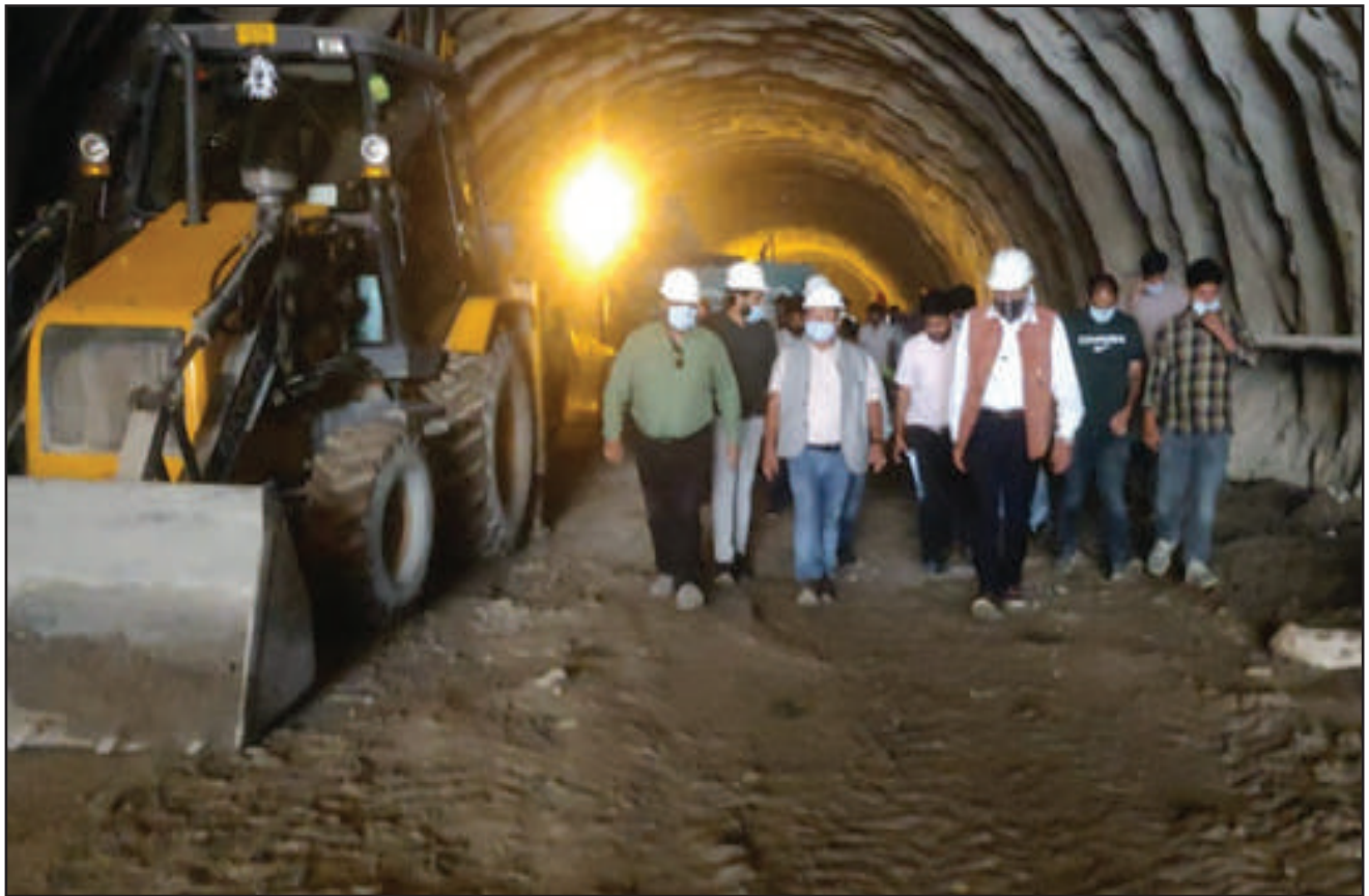
83rd Tunnel, Jammu & Kashmir
