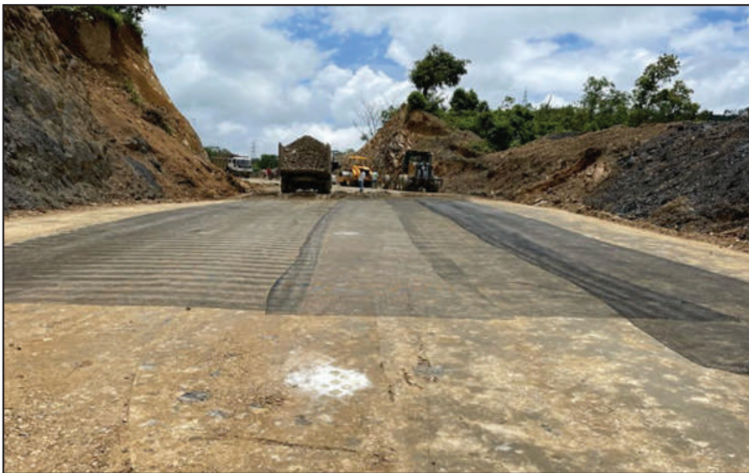
Kohima Bypass Road (Nagaland)
