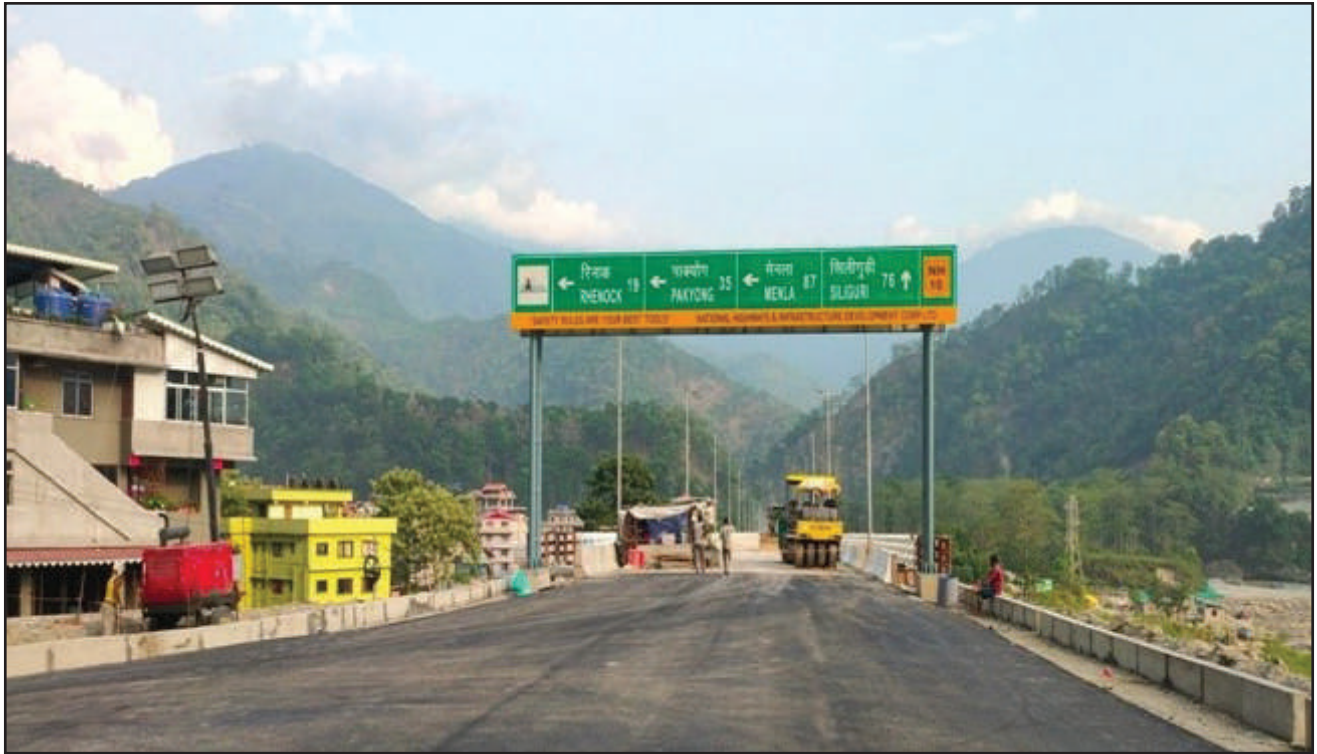
Rangpo Viaduct Connecting Sikkim with West Bengal.
