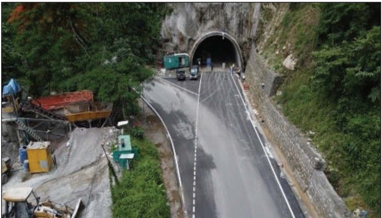
Chisopani Traffic Tunnel - Sikkim.
