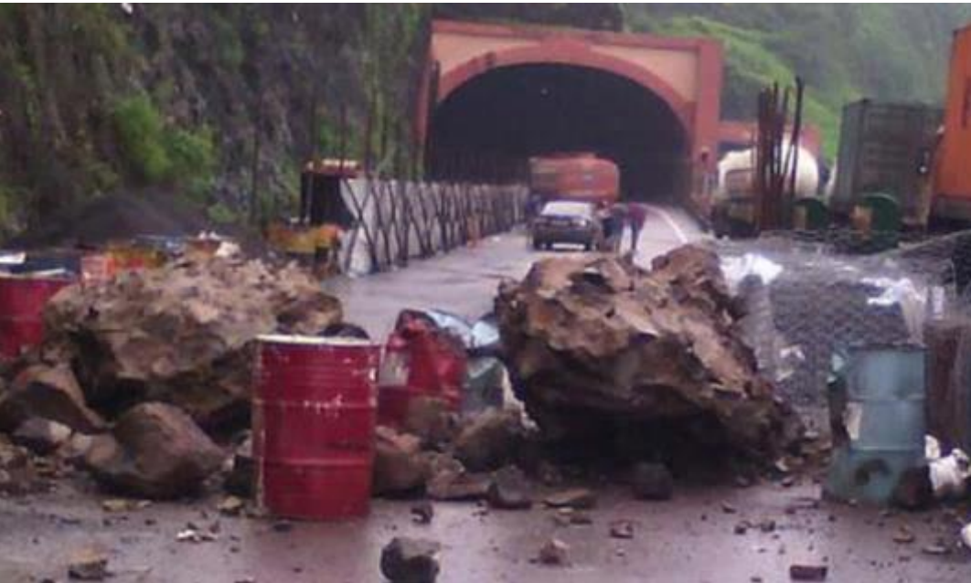
Photograph showing the rock slide near Khandala tunnel (Mumbai corridor) (source: NDTV news)
