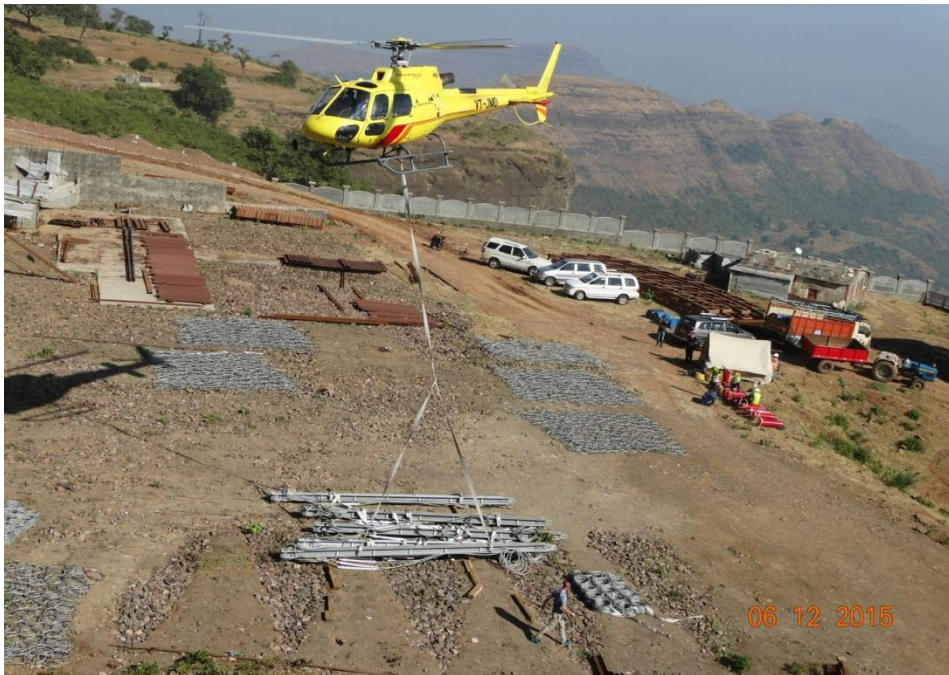
Helicopter waiting in Helipad to take off with barrier components
