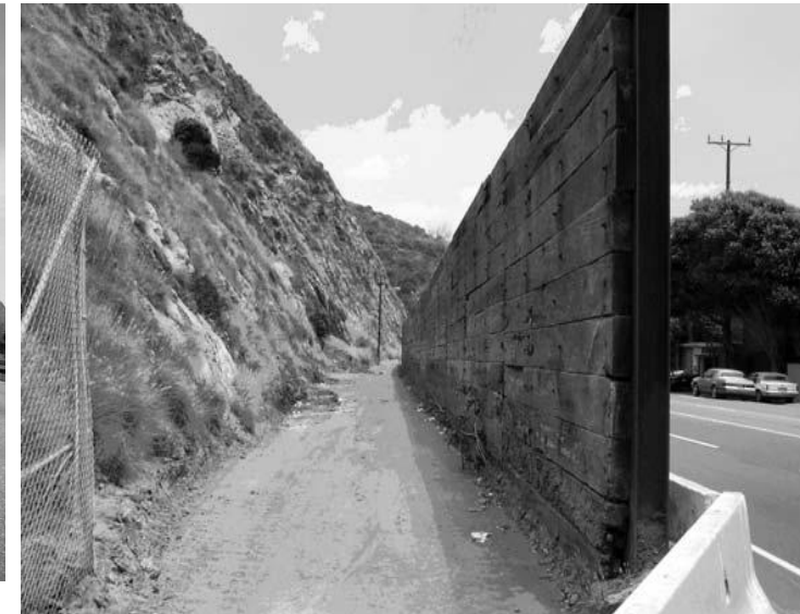
Timber Soldier-pile walls
