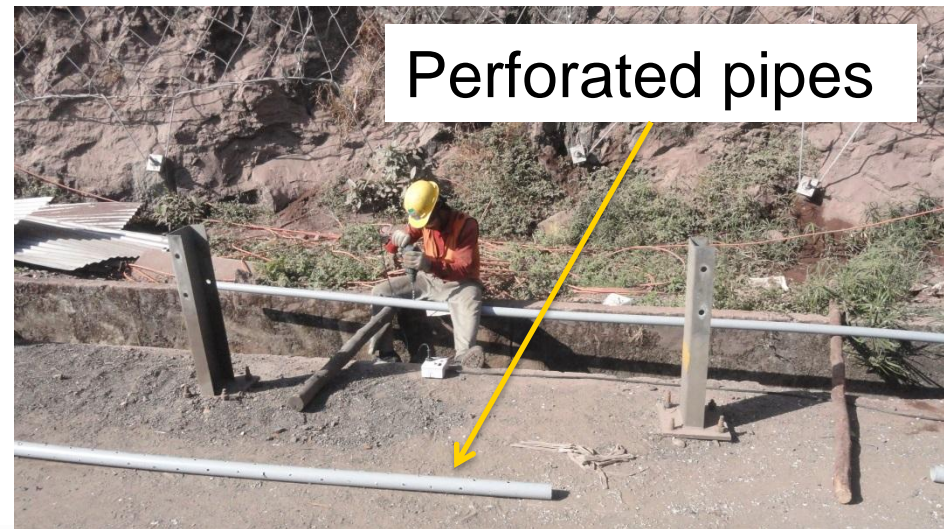
Rockfall Mitigation Measures
