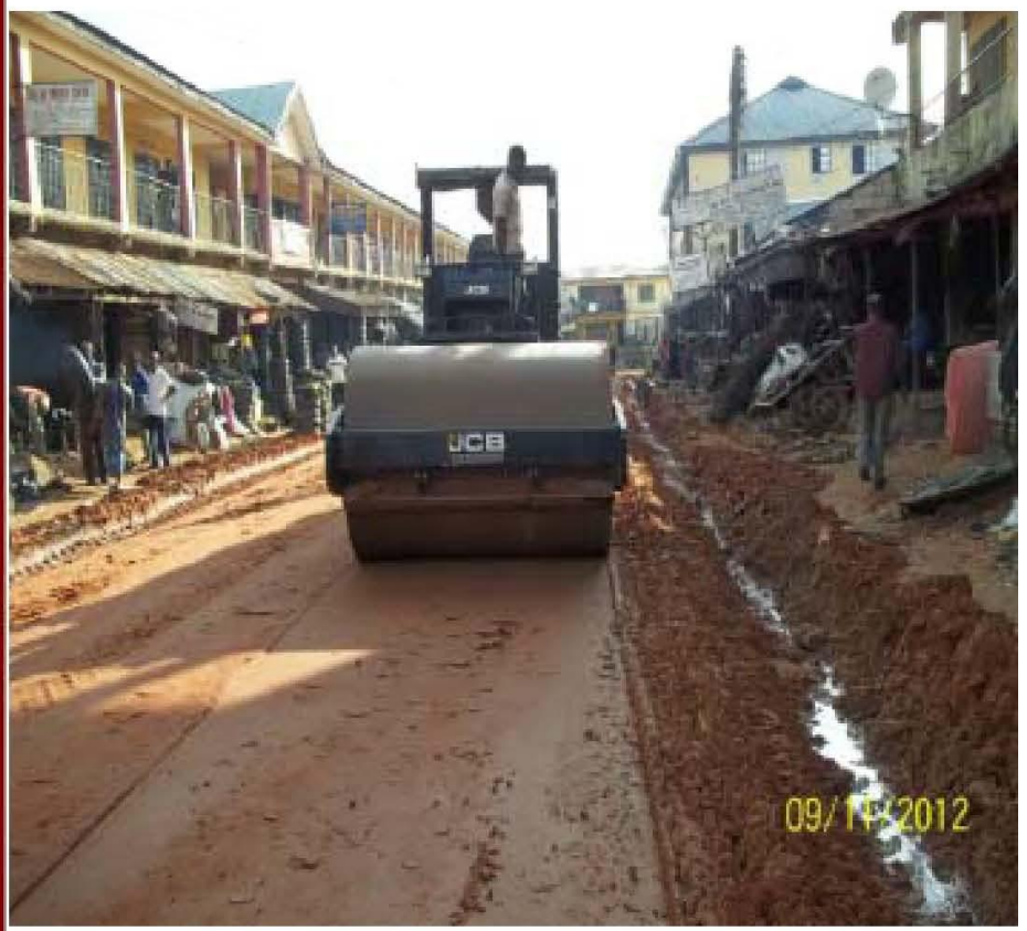
Finishing with a vibratory steel-wheeled roller
