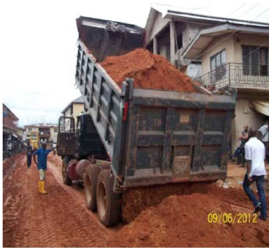
Additional borrow material to elevate road for drainage
