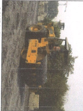
COMPACTION OF SOIL BEYOND 1.5m WIDE ZONE FROM PANELS (FIGURE - 37)
