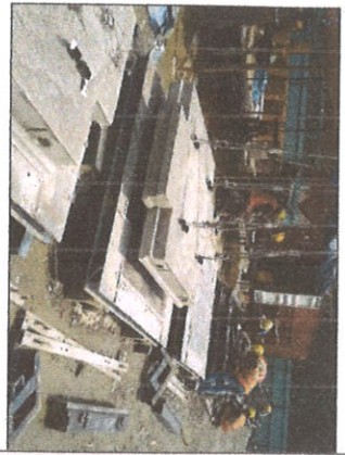
FIGURE - 18) LIFTING OF PANELS NOTE: USE OF FOUR POINT SLING IS MANDATORY TO AVOID DIAGONAL CRACKING)
