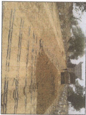
LAYING OF PET POLYMERIC STRIP AND BACKFILL & WINDROWING (FIGURE - 36)
