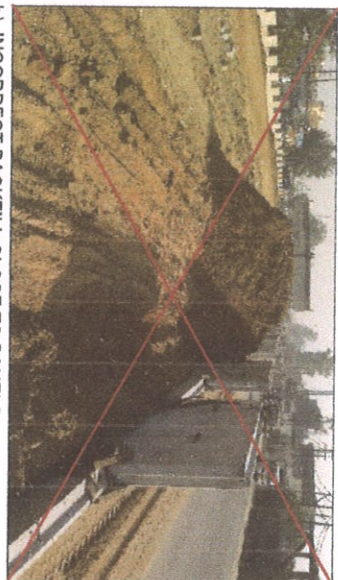
b). INCORRECT BACKFILL CLOSE TO PANELS
