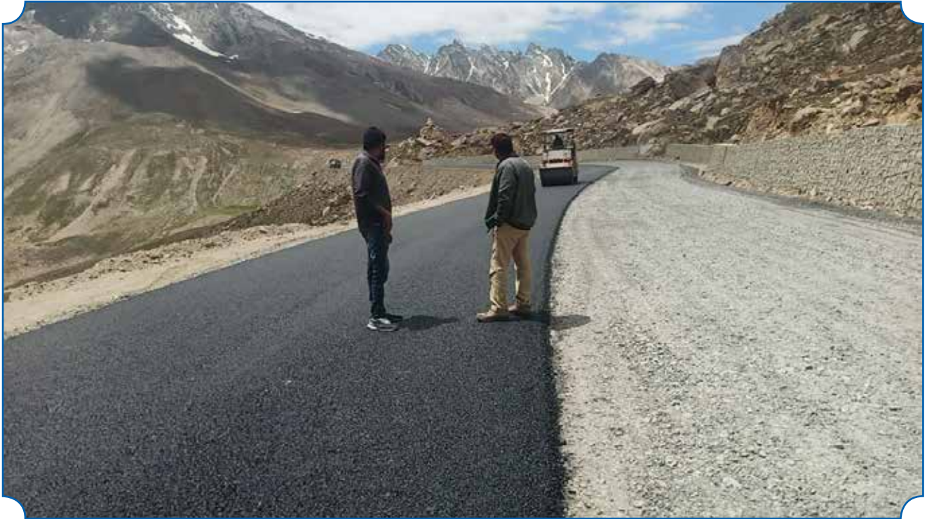
A View of Kargil-Zaskar Road Ladakh Pkg-VII DBM rolling work in progress at 155+000, Ladakh
