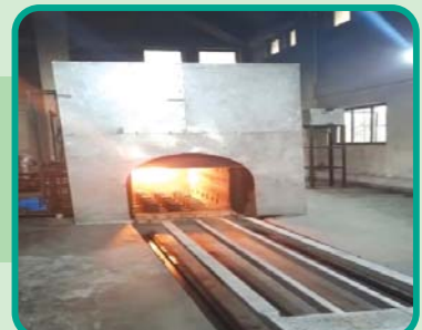
Replacement of 2 nd Furnace of the Shillong Electric Crematorium, Shillong, Meghalaya
