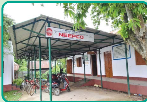
Construction of Cycle Stand at Taranagar High School, Mohanpur, Tripura (West), Tripura
