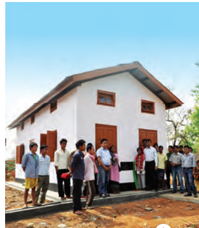
Community hall at Langmeklu village, Umrongso, Assam
