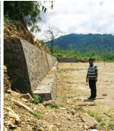
Construction of playground with protection wall at Kimi Village
