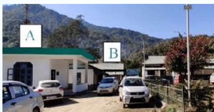
Construction of the Community Health Centre (CHC), Yazali, Arunachal Pradesh
