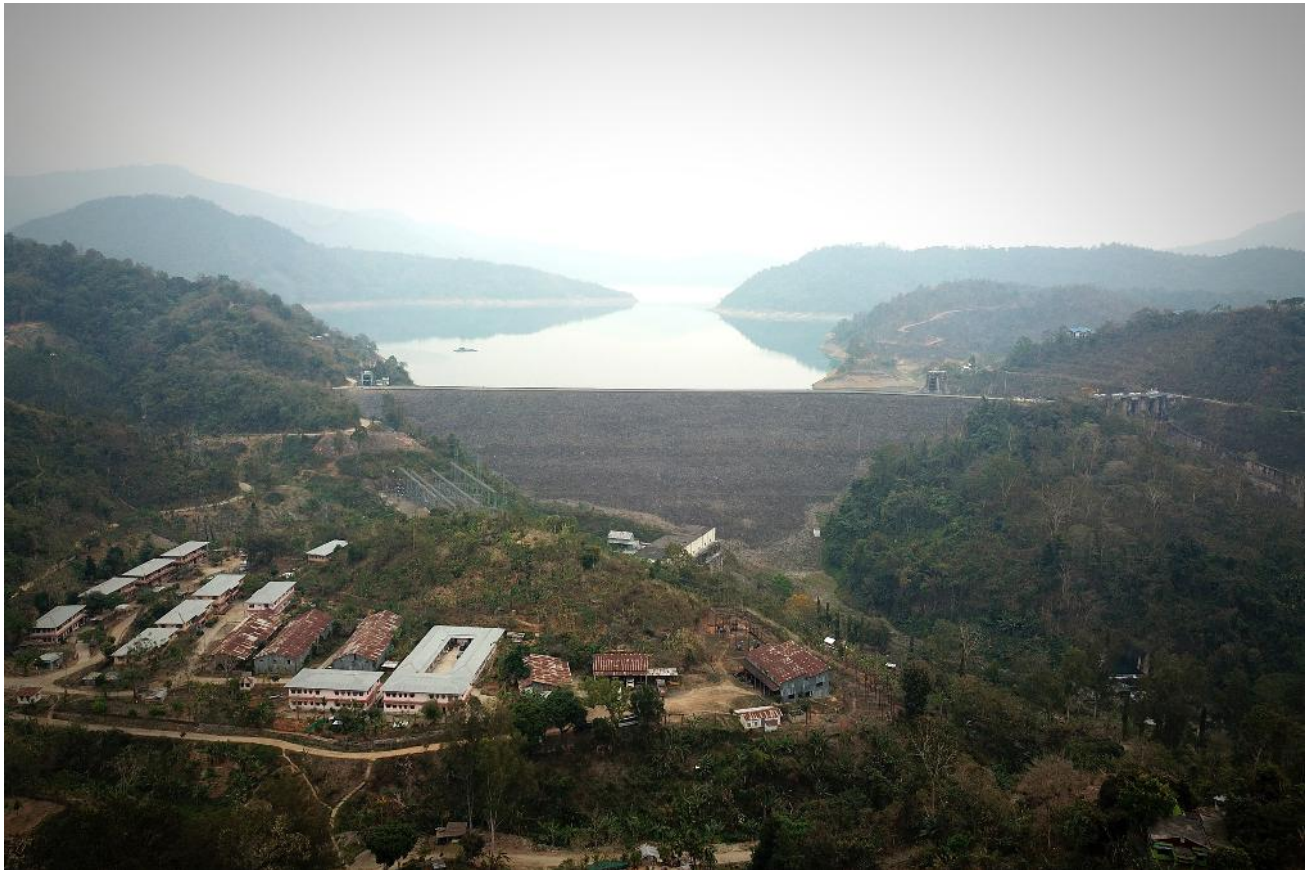
Doyang Hydro Project
