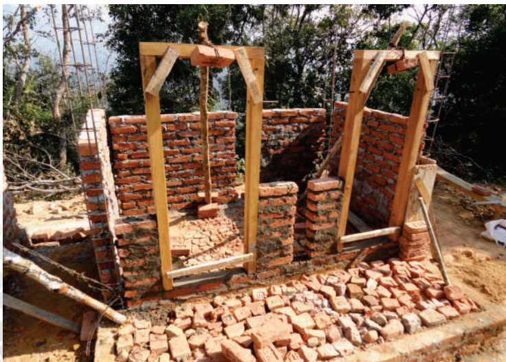
School toilets in progress at wokha Nagaland
