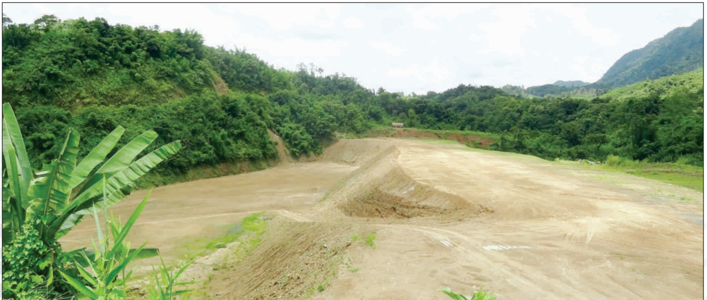
Upper Cofferdam, Tuirial Hydro Electric Project
