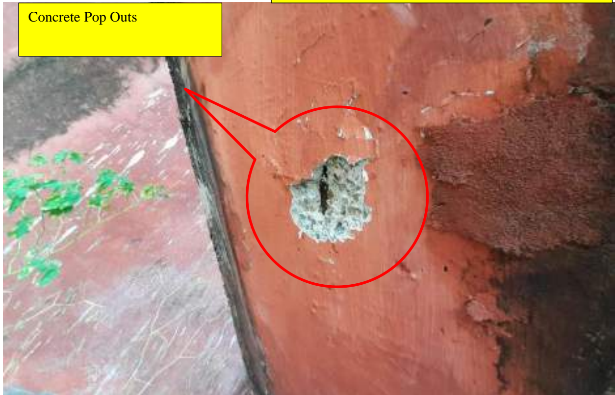
Swelling of concrete and map cracking patterns are also observed
