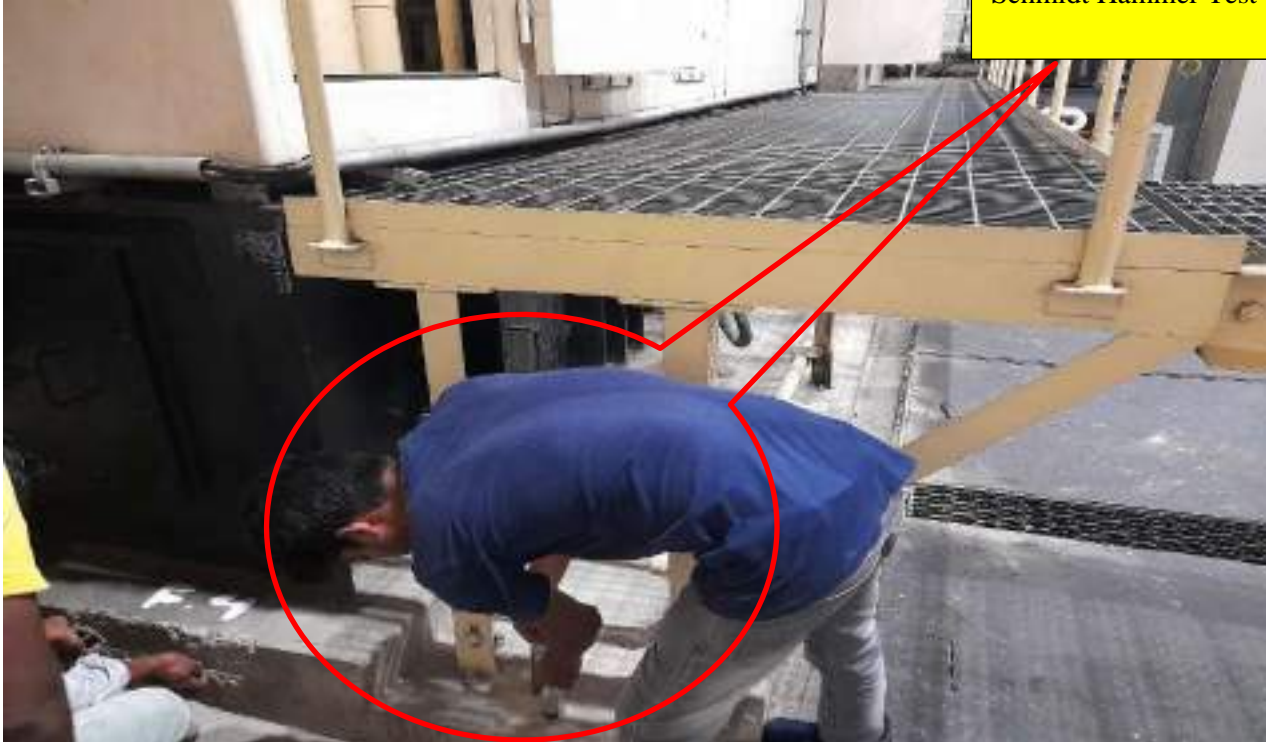
Ultrasonic pulse velocity Test of concrete
