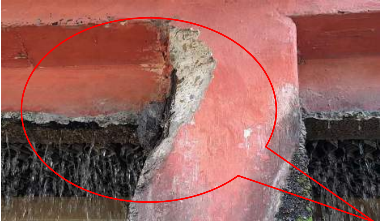
Spalling of concrete due to reinforcement corrosion
