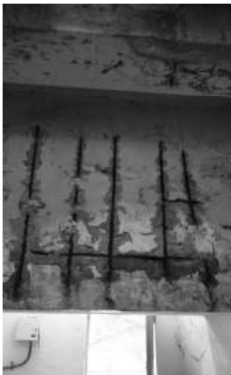
CW pump house civil structure
