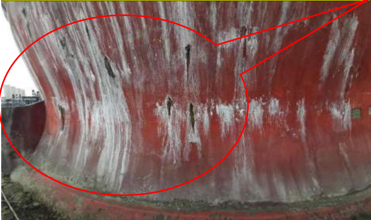
Severe calcium leaching is observed
