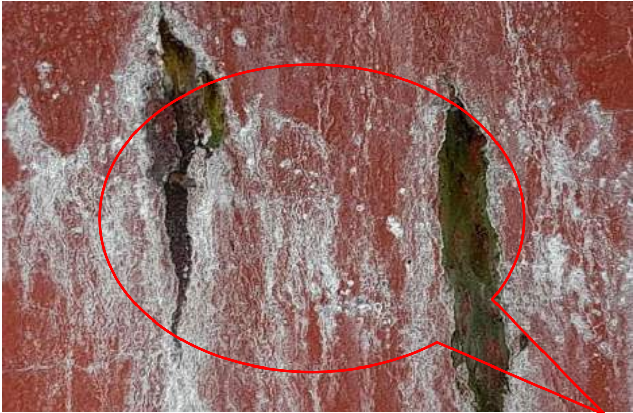
Severe calcium leaching is observed
