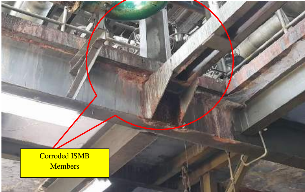
Pitting corrosion due to water leakage
