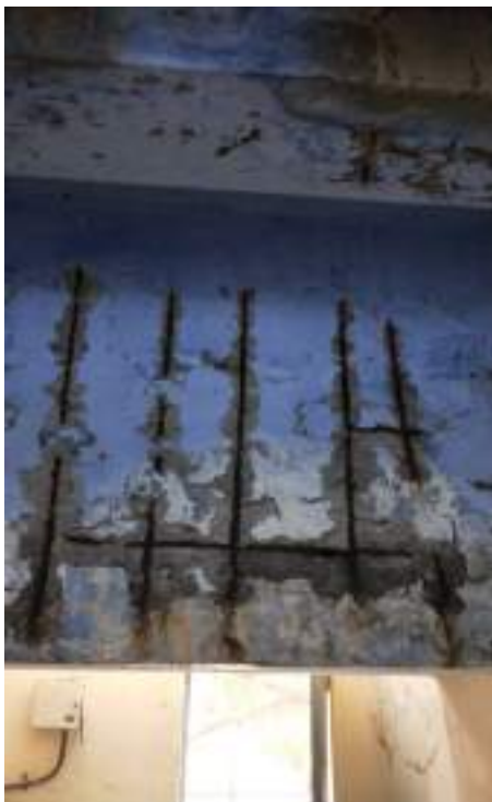
CW pump house civil structure
