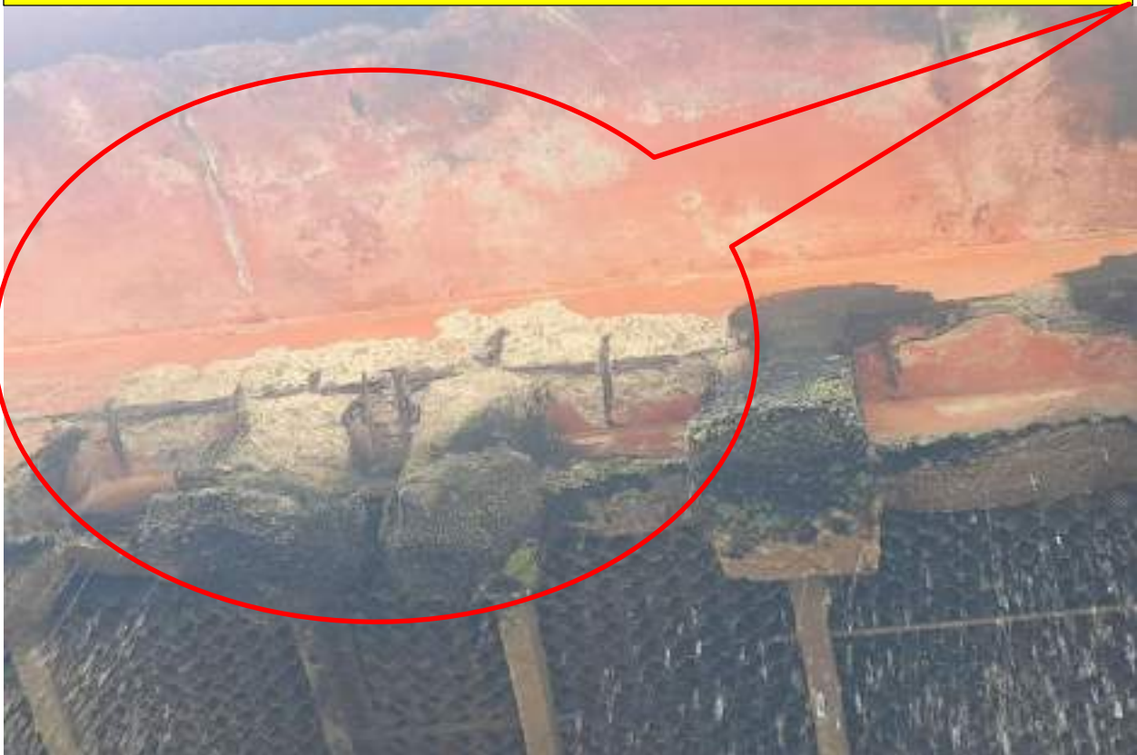
Spalling of concrete due to reinforcement corrosion
